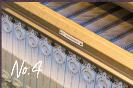
Plant 134 Surface Water Treatment Plant Membrane Replacement
