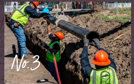
Water Main Replacements
