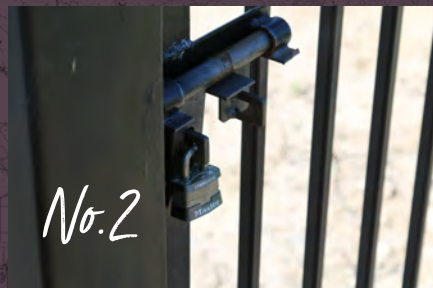
Plant 134 Security Fence Upgrade
