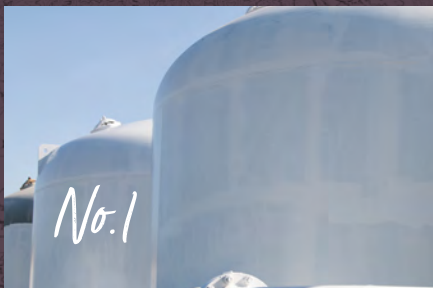
Plant 108 Tank Mixer Addition
