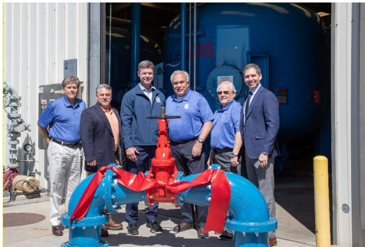
Photo Caption: East Valley Water District's Board of Directors and General Manager/CEO turn the valve on the Surface Water Treatment Plant enhancement. Left to right: David E. Smith, Governing Board Member; James Morales Jr., Vice Chairman of the Board; Michael Moore, General Manager/CEO; Phillip R. Goodrich, Chairman of the Board; Ronald L. Coats, Governing Board Member; Chris Carrillo, Governing Board Member.
